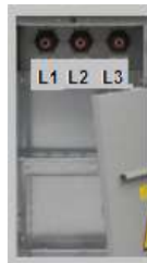
Figure 26 – Marking of the phases
